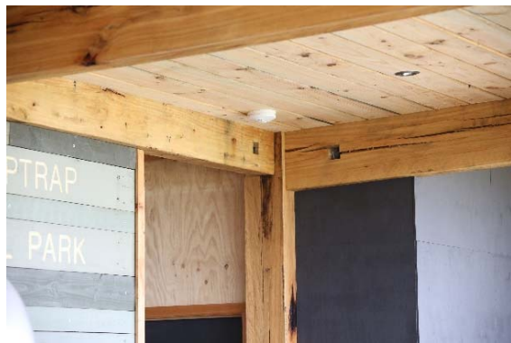
Figure 24: Details of the beam and post structure: the square hole allows the joining bolt to be tightened in situ .
