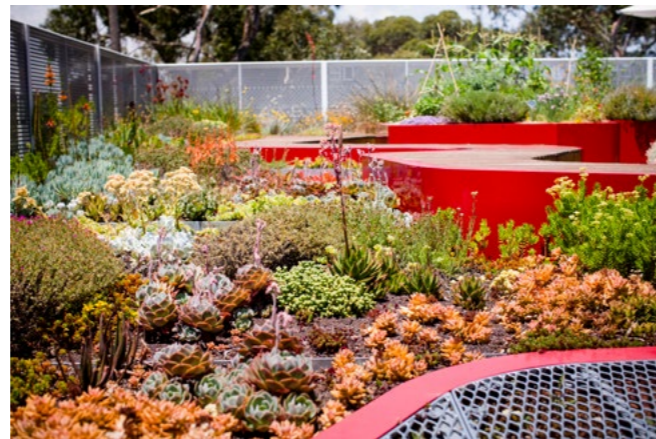
Figure 5.1 Burnley Demonstration Green Roof showing substrate depths and irrigation of different zones. Plants in this case study are found in the 10, 15 and 20 cm unirrigated scoria beds zones 1-3. Images: University of Melbourne.
