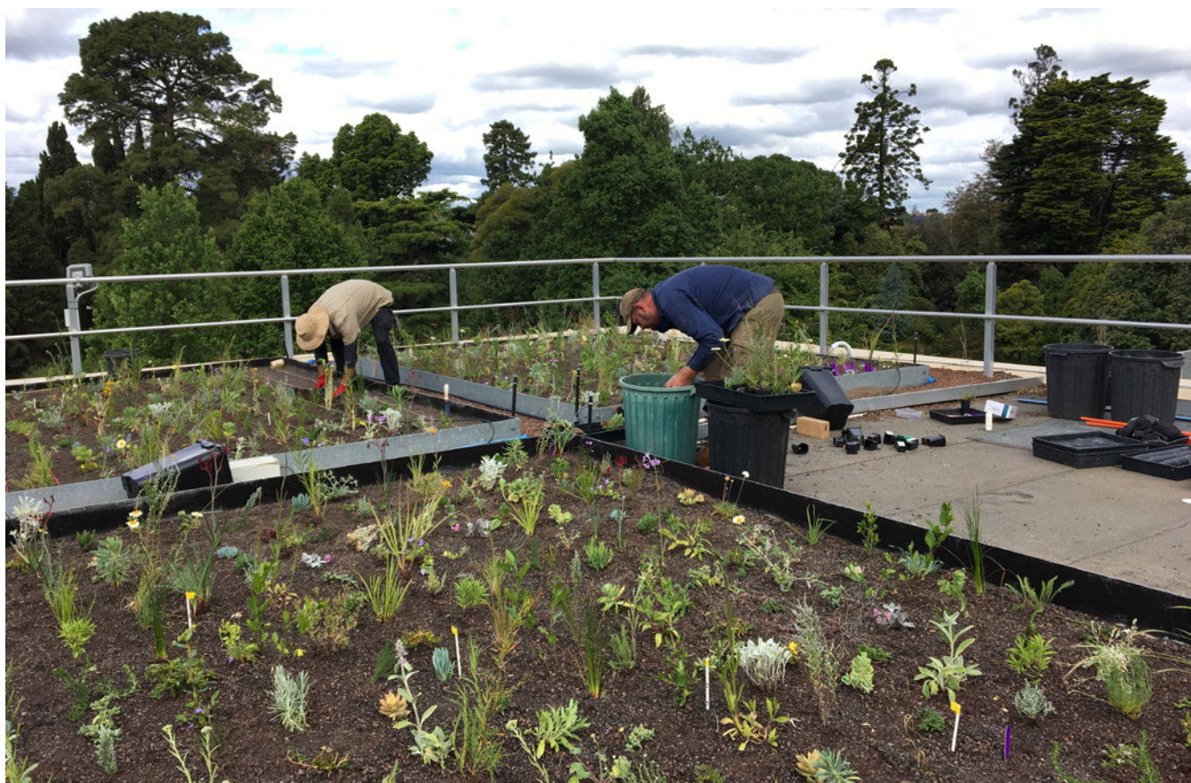
Regular weeding is an essential maintenance task for achieving designed vegetation outcomes and green roof function. Burnley research green roof, University of Melbourne. Image: R. Bathgate
