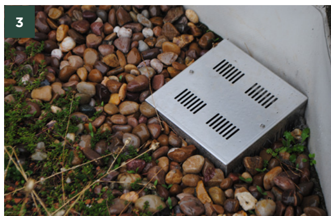
Drainage is a critical component of green roof infrastructure. Drainage areas should be free of any vegetation and plant debris, with regular monitoring of drainage pits, inspection chambers, gutters, flashing and downpipes. Images: 1. & 3. J. Rayner, 2. E. Snodgrass
