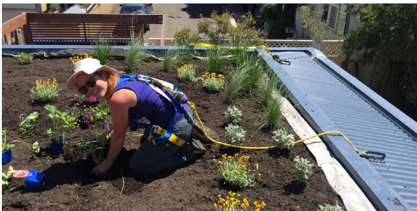
Fall arrest systems require dedicated personal protective equipment (PPE) to protect an individual from injury in the event of a fall from a roof and include use of a full body harness, lanyard, rope lines and secure roof anchor points. Image: S. Hardgrove
