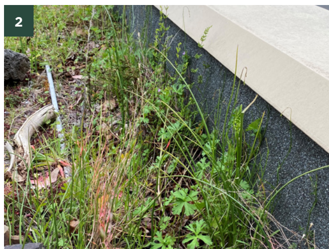
1. Woody weeds can be particularly problematic on green roof as roots can penetrate underlying layers, requiring care when removing to avoid further damage and removal of substrate. Image: E. Snodgrass 2. Regular weeding of the non-vegetated perimeter on green roofs ensures that drainage functions properly and reduces further problems caused by weed ingress into drains and flashing. Image: J. Rayner
