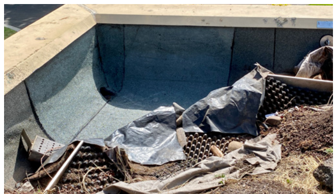
Drainage problems on this corner of the green roof took many years to be resolved (Nov 2020).
