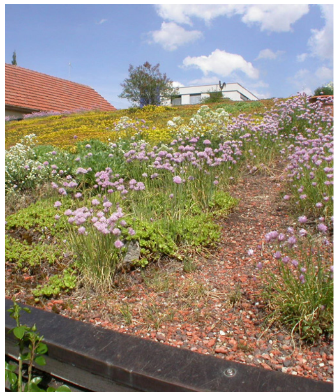
Low-growing succulents are the main plant type on this shallow green roof in Stuttgart, Germany. Image: J. Rayner
