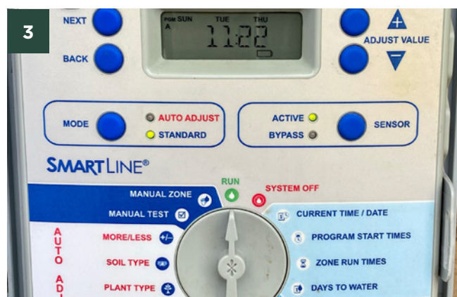
Microspray and drip systems are the most widely used irrigation systems on green roofs across Australia. 1. Inline drippers using purple pipe (non-potable water source) on the Burnley demonstration green roof. 2. Microspray emitters. 3. Irrigation controllers are critical in managing irrigation systems. Images: 1. & 3. J. Rayner, 2. E. Snodgrass
