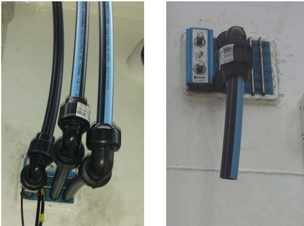
*Figure 3: Penetration through the wall of the container for detector plumbing and connection to the main inlet line (left) and exhaust line (right).*
