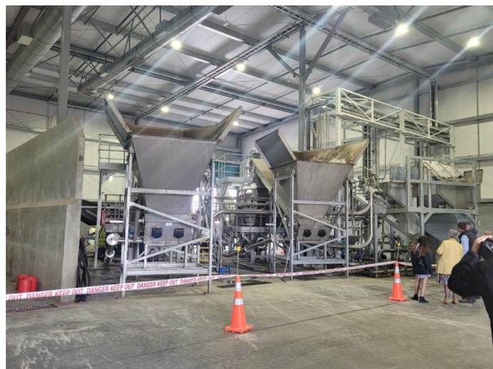
Figure 46: Sorting hoppers which receive and filter organic waste streams at Ecogas' Reporoa plant.
