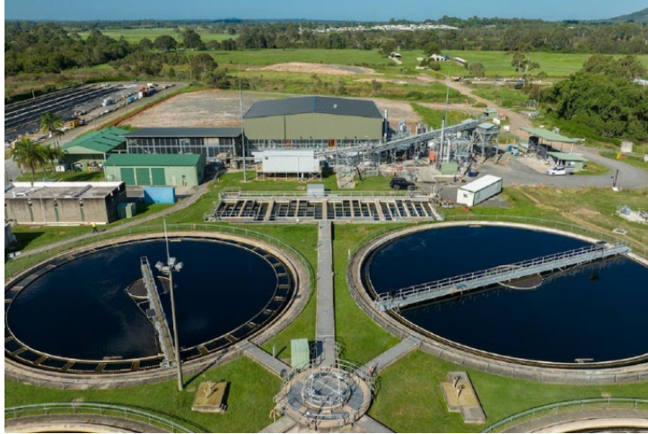
Pyrocal's gasification facility at Loganholme (background) next to two wastewater treatment ponds (foreground). Image credit: Pyrocal.
