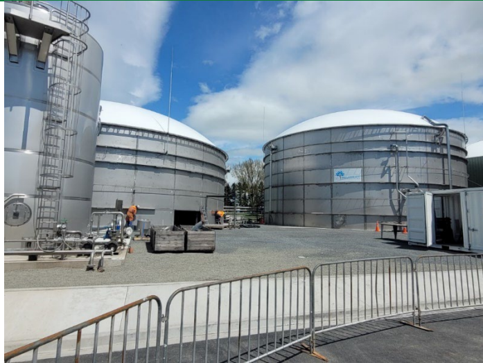
The digester tanks at Reporoa which hold up to 3,500,000 litres of organic waste. Methane rises to the top of the tanks and are captured using a hose system.
