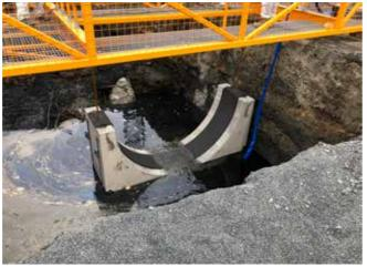
Concrete cradle for pipe support being lowered into place.
