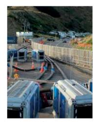
The six 8" BBA BA180 auto prime dewatering and sewer bypass pumps on site at Moa Point.
