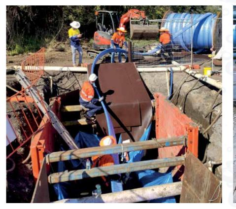
The small installation footprint is small. Installation of 800 metres DN 300 Primus Line in a sewer rising main though an existing maintenance chamber. Primus Line can also be used to renovate vertical pipelines.
