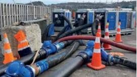
The Netherlands-designed pumps, overpumped 928 million litres of wastewater during the project.
