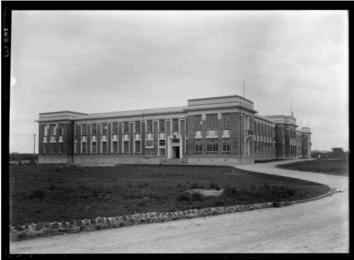
The 'red' building, as it was known to some trainees, was erected in 1925 and demolished in 1976. Henry Winklemann, Auckland Teachers Training College, Epsom, 1926 , Auckland Libraries Heritage Collections 1-W0681.
