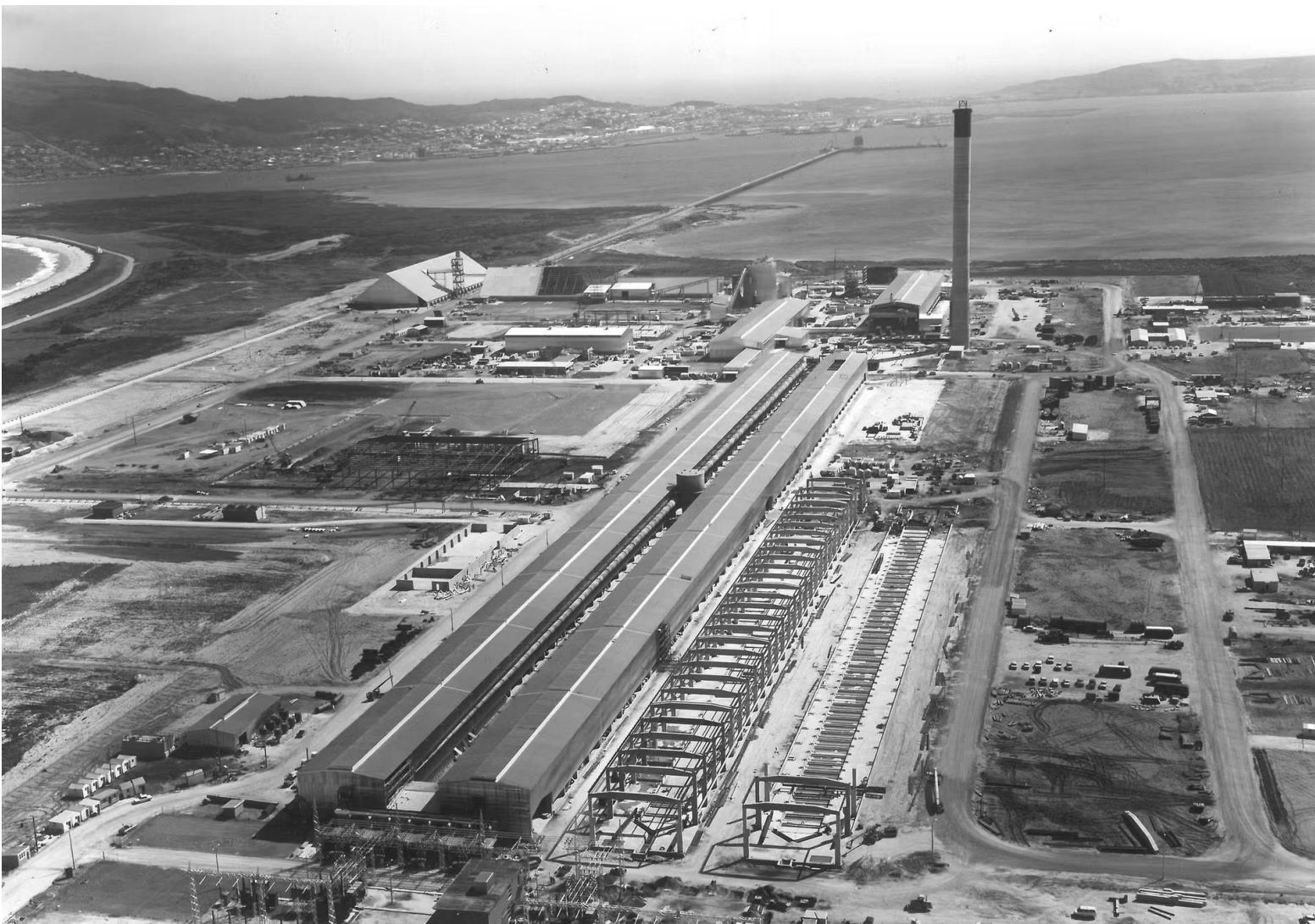
Construction of Tiwai Point Smelter early 70's – from the NZAS website, accessed 27/01/26
