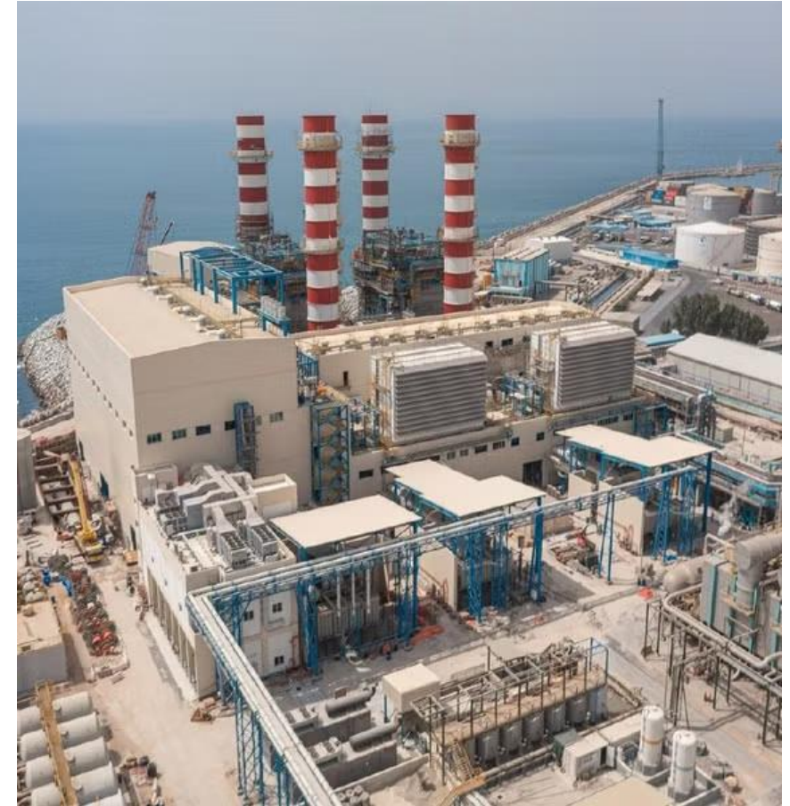
Alba's Power Station 5 ..... a new 680.9MW combined-cycle power plant - Mitsubishi Power
