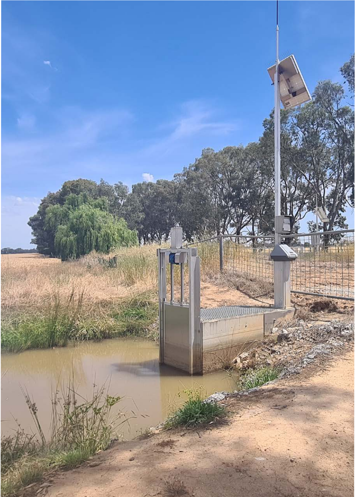
Figure 3: Water meter with telemetry, southern NSW 2020.
